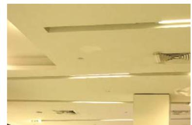
Recessed light troffers created with Fastcap: quick, straight and sturdy for fixing lighting components
